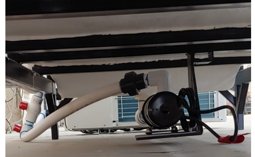
FilterMax pump located under the tank
